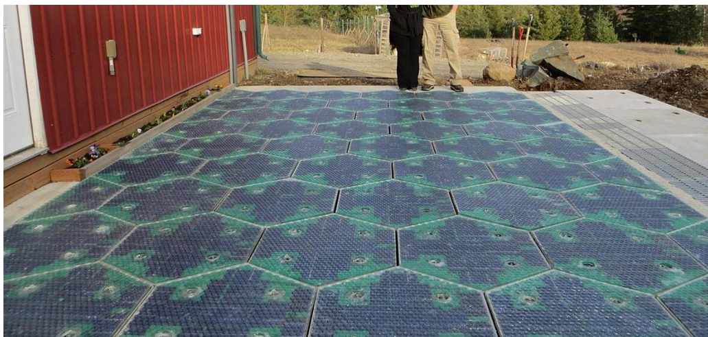
Figure 2 The Solar Roadways parking-lot prototype in Idaho, USA (interlocking solar panels in the pavement).
