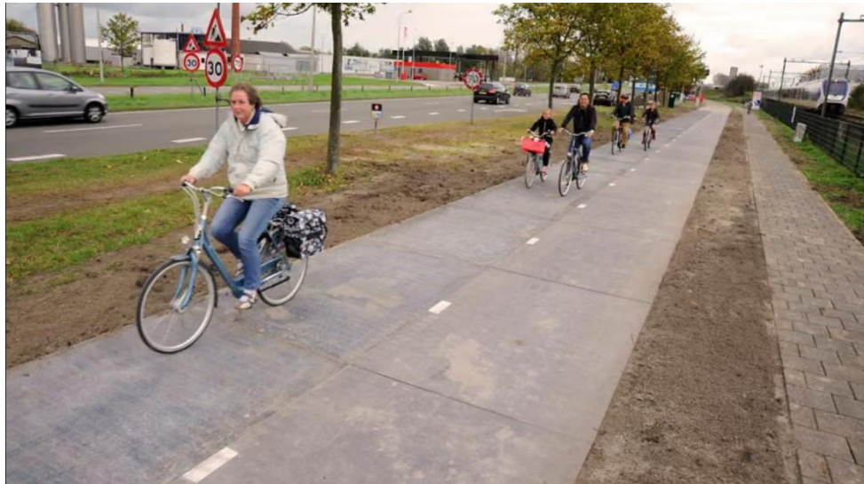
Figure 1 The SolaRoad solar bike lane in Krommenie, Netherlands (solar panels embedded in pavement under a translucent protective layer) (Oltermann, P., 2014)
